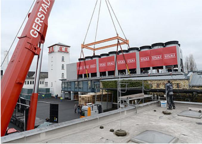
The chilling system was manufactured in STULZ's Hamburg factory and delivered straight to the construction site.
